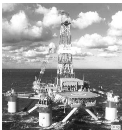
Offshore structures require strict notch toughness in order to endure operations in harsh weather and roaring waves.
