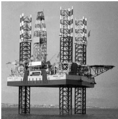
Jack-up rig is a typical construction that requires high performance filler metals with high impact toughness and low crack susceptibility. (Photo courtesy of Kansai Design Co., Ltd., Japan)
