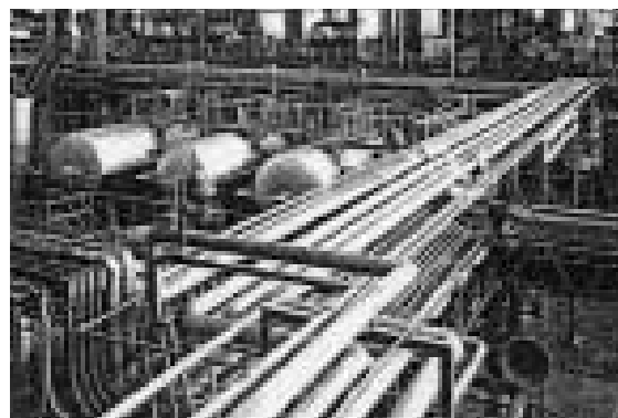
Fig. 1. TGS-2CML is more suitable for welding process-piping joints subject to short-time postweld heat treatment - thus lower temper parameter.
