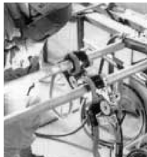
Fig. 2. An automatic TIG welding process of tube-to-tube butt joints
