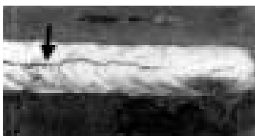
Fig. 1 A longitudinal hot crack appearing on the surface of a weld metal by SMAW (left)
