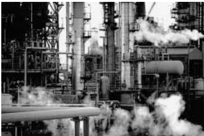
Photo 1. A refinery is composed of a variety of sophisticated equipment such as reactors, towers, heat exchangers, and pipelines.
