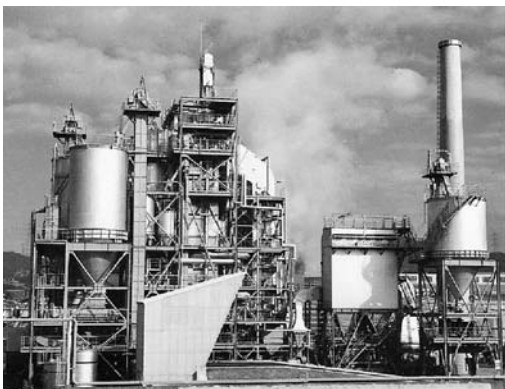
Heat-resistant low-alloy steel is a main material for coal firing power plants
