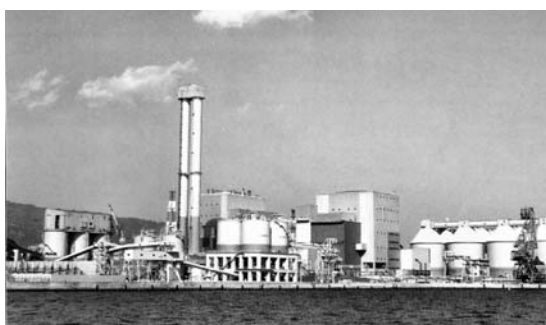
2.25Cr-1Mo steel is an indispensable material in a coal-fired power plant (Kobe Steel's power plant)
